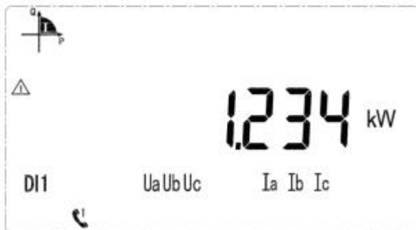
Current total power is 1.234kW
